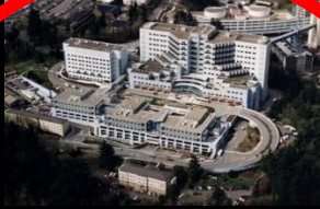
Auditory Rehabilitation (Portland, OR)
